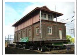
An Australian first - the relocation of the Hornsby Signal Box in one piece
